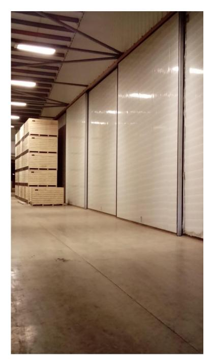
Figure 2: Doors across stack ends to avoid 'backfill'
